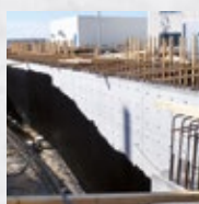
External basement waterproofing
