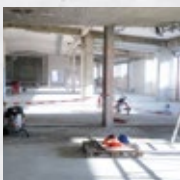
Restoration of support beams
