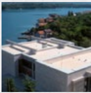
Liquid roof waterproofing
