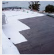
Waterproofing on bitumen
