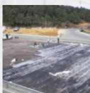
Floor slab waterproofing
