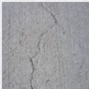
Penetrates into very fine cracks
