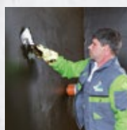
Waterproofing against Radon
