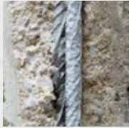
Corrosion protection (coating)
