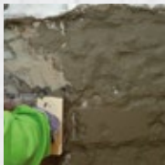
Internal basement waterproofing
