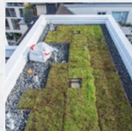
Under ballast / green roofs
